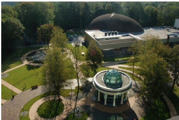
Figure 3. Unique architecture in Druskininkai (Lithuania) as compact, safety and polyfunctional modern public urban structure
